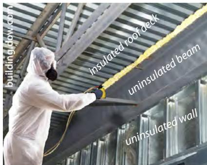
**Sealing the roof deck:** Seal the roof wall junction with spray foam. Insulate the walls above the suspended ceiling. Insulate the roof deck if there's no insulation on top of the roof deck.
