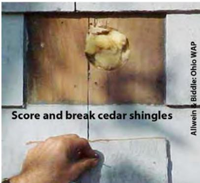
**Score and break a shingle:** If the shingles are flexible, you may be able to remove nails. However, usually you must score and break the shingle, and then later face-nail it back in place.
