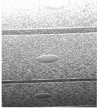
**Blowing through the ceiling:** The contractor pushes the fill-tube into the cavity and out near the edge of the roof. The holes are drilled in a straight line for appearance sake.
