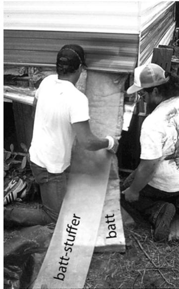
**Batt-stuffing walls:** Installers use a flexible plastic plank to stuff a fiberglass batt into an empty or partially filled wall cavity. Installers remove screws from the bottom of the siding. Joints between sheets usually remain locked together during batt-stuffing.
