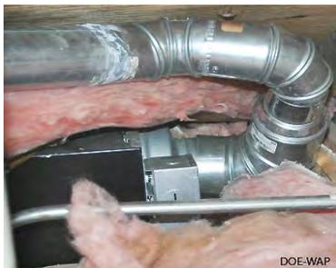
**Wrong-way fan orientation:** Turning the air stream 180 degrees substantially reduces airflow.
