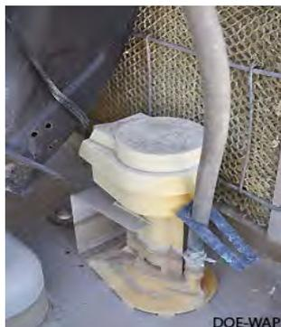
**Pump delivers water to distribution tubes:** Clean the reservoir and the pump of dirt and scale.
