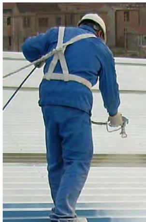
Bare galvanized steel and aluminum aren't nearly as cool as white roofing. Those shiny metals reflect solar heat well, but they don't emit heat effectively so they tend to heat up, resulting in SRIs in the 40s for bare galvanized steel and in the 70s for bare aluminum.
