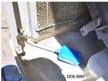
**Float controls water supply:** Make sure that the float shuts the water off completely when the reservoir is full.
