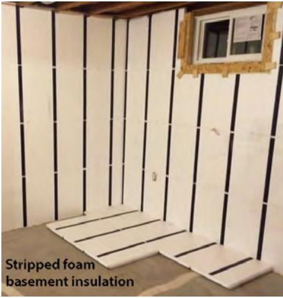
**Installing striped foam:** Installers glue and screw the foam sheets to the masonry wall and concrete slab. Then they glue drywall to the foam and screw the drywall to the strips.
