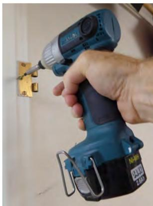
**Solutions for door sagging:** Bend the hinge knuckles slightly, drive a long screw into the hinge, and/or drive another long screw into the jamb above the hinge. Experience will tell you which solution works in each particular case.
