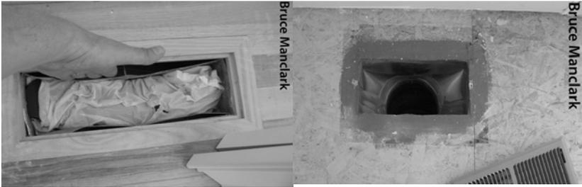
**Sealing register boots:** Seal between the boot and floor. Seal joints inside the boot.
