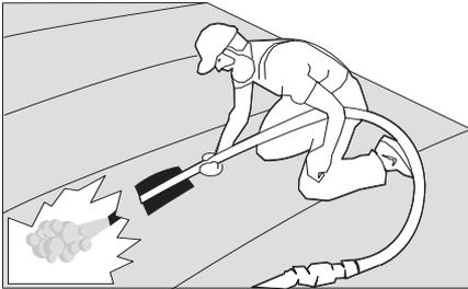
**Roof-top insulation:** Blowing fiberglass insulation through the roof top is effective at achieving good coverage and density on almost any metal roof. Use walk boards to avoid damaging the roof.
