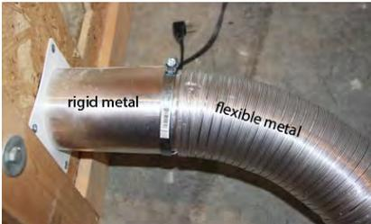
**Vent and termination:** Use rigid metal vent pipe if at all possible. Or use flexible metal vent and not foil vent when flexibility is required.
